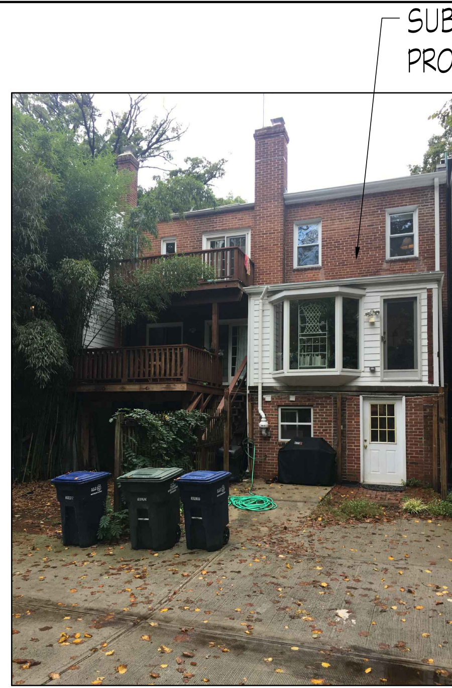
2 VIEW OF REAR LOOKING WEST TO PROPERTY TO THE SOUTH, LOT 76
